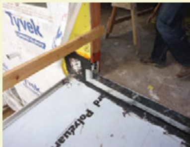
PHOTO 4 Membrane Waterproofing. Additional metal flashing is installed over the waterproofing that is stripped into the pan flashed balcony door opening. This additional metal flashing protects the membrane waterproofing at the door opening.
