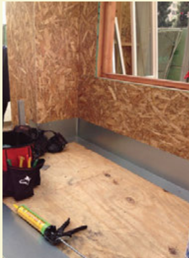
PHOTO 2 Metal Angle. Note the use of plywood as the balcony deck surface. Plywood and engineered wood deck sheathing are typically both used interchangeably. However, adhesion of membrane waterproofing to engineered wood deck sheathing tends to be more difficult and primers become key to successful adhesion. PHOTO 3 Pan Flashing of Balcony Door. Note the back dam and end dam of the flashing for the balcony door. The back dam support for the pan flashing has not yet been installed. The back dam support protects the upstand of the back dam during the construction process.
