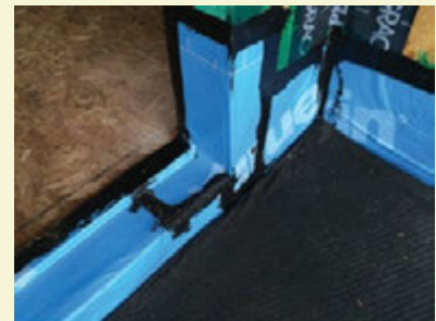
PHOTO 2 Metal Angle. Note the use of plywood as the balcony deck surface. Plywood and engineered wood deck sheathing are typically both used interchangeably. However, adhesion of membrane waterproofing to engineered wood deck sheathing tends to be more difficult and primers become key to successful adhesion. PHOTO 3 Pan Flashing of Balcony Door. Note the back dam and end dam of the flashing for the balcony door. The back dam support for the pan flashing has not yet been installed. The back dam support protects the upstand of the back dam during the construction process.
