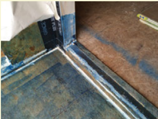
PHOTO 1 Sealant Joint. A sealant joint is installed at the perimeter of the balcony deck where it intersects the exterior wall. Note the primer application on engineered wood deck sheathing and the OSB wall sheathing. The primer's function is to facilitate adhesion of the waterproofing membrane. Also note the back dam support for the yet to be installed pan flashing in the rough opening for the balcony door.
