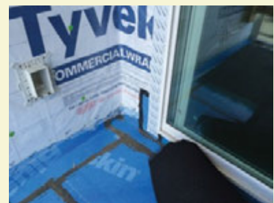
PHOTO 5 Drainage Mat. Membrane waterproofing is stripped into the pan flashed balcony door opening. Note the drainage mat installed over the top of the membrane waterproofing. Also note the mastic application sealing the vertical portion of the balcony deck waterproofing membrane to the wall sheathing.
