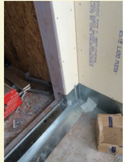
PHOTO 2 Metal Angle. Note the use of plywood as the balcony deck surface. Plywood and engineered wood deck sheathing are typically both used interchangeably. However, adhesion of membrane waterproofing to engineered wood deck sheathing tends to be more difficult and primers become key to successful adhesion. PHOTO 3 Pan Flashing of Balcony Door. Note the back dam and end dam of the flashing for the balcony door. The back dam support for the pan flashing has not yet been installed. The back dam support protects the upstand of the back dam during the construction process.
